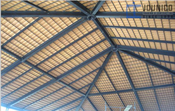
BRICK ROOFING- HABBOUCH
