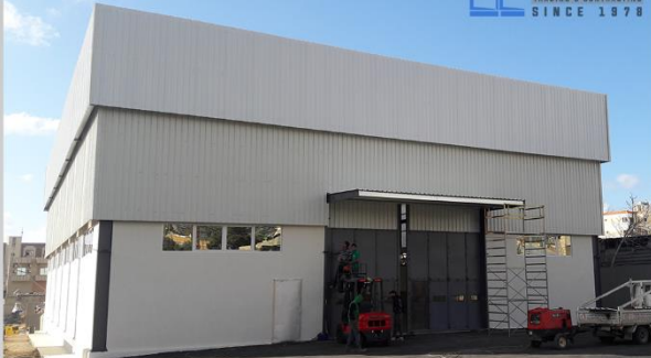
BREAKER - KAEEN GROUP - GHAZIEH
